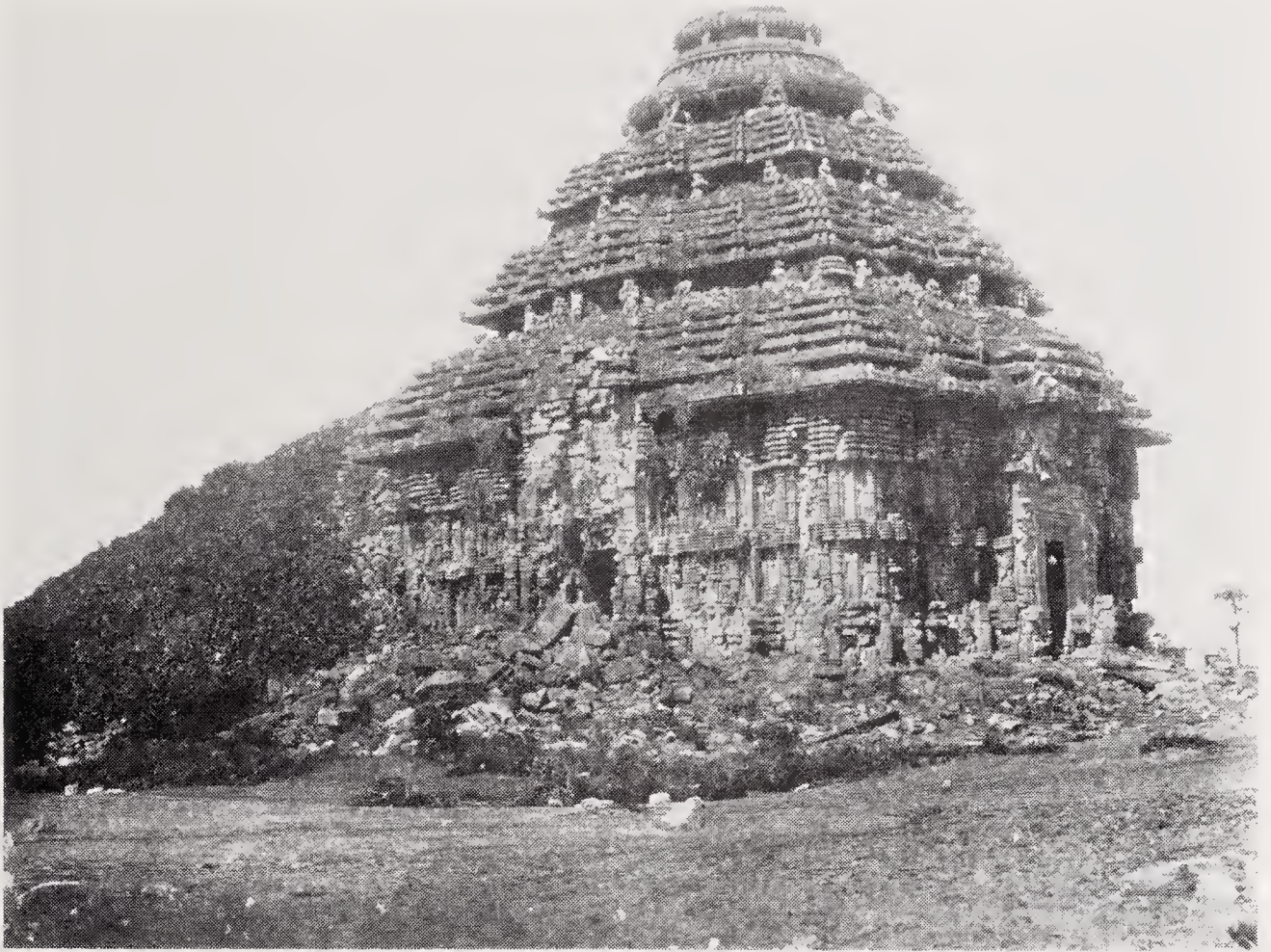
View of the Sun temple before repair, ASI.
